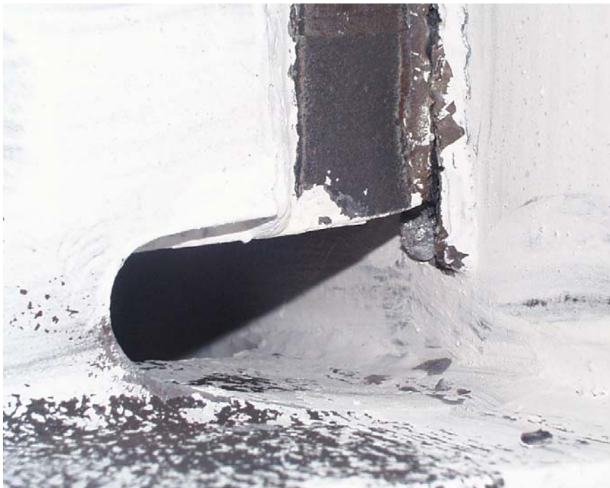
(e) Bottom edge of shear tab weld (after test)
