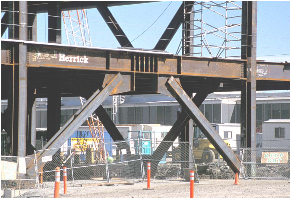
Figure 1.1 Example of recently constructed EBF
