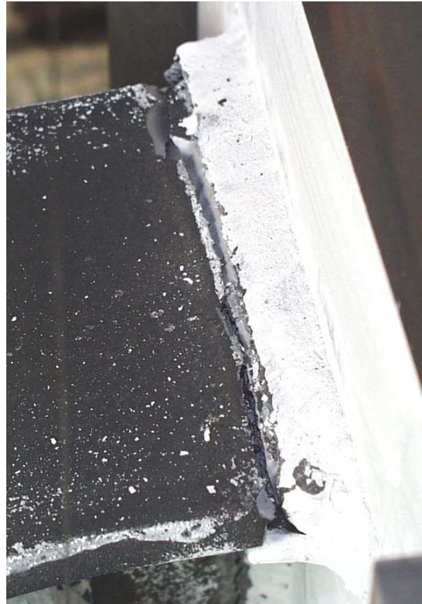
(b) Fractured link top flange after test
