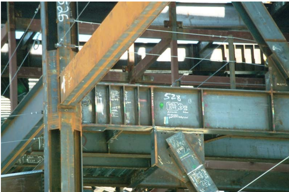
Figure 1.2 Example of link-to-column connection
