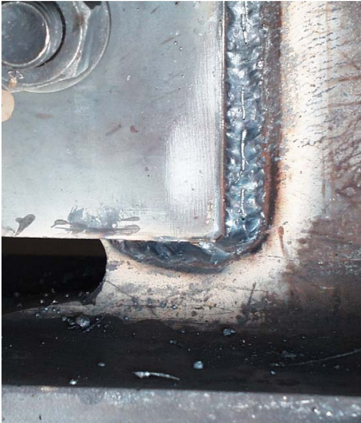
(a) FFS shear tab bottom
